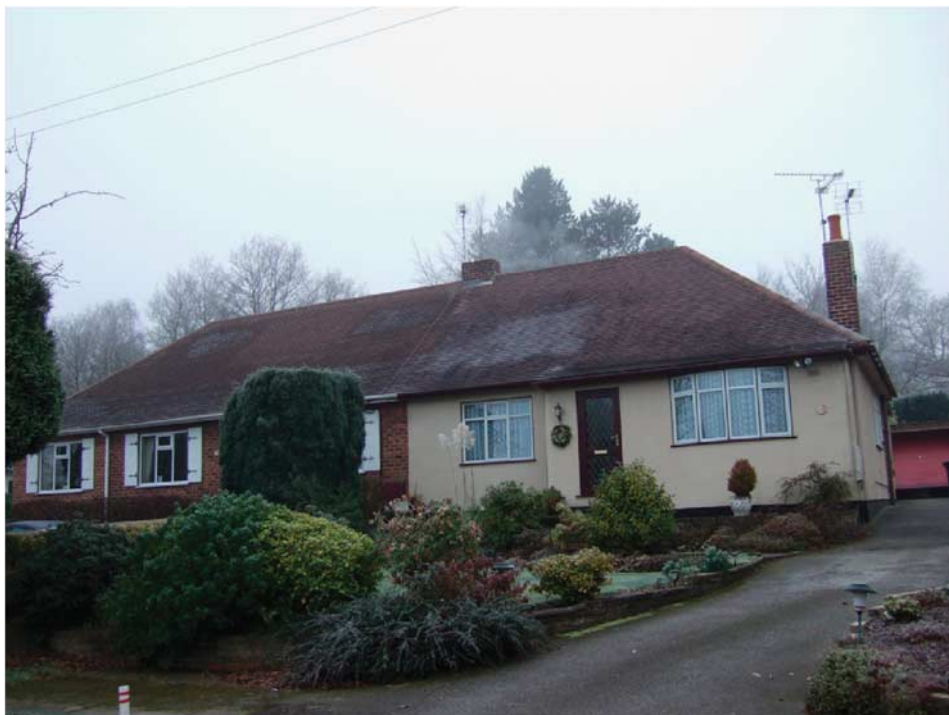
Figure 4: A pair of originally prefabricated semi-detached properties dating from the late 1950s which have evolved differently.
