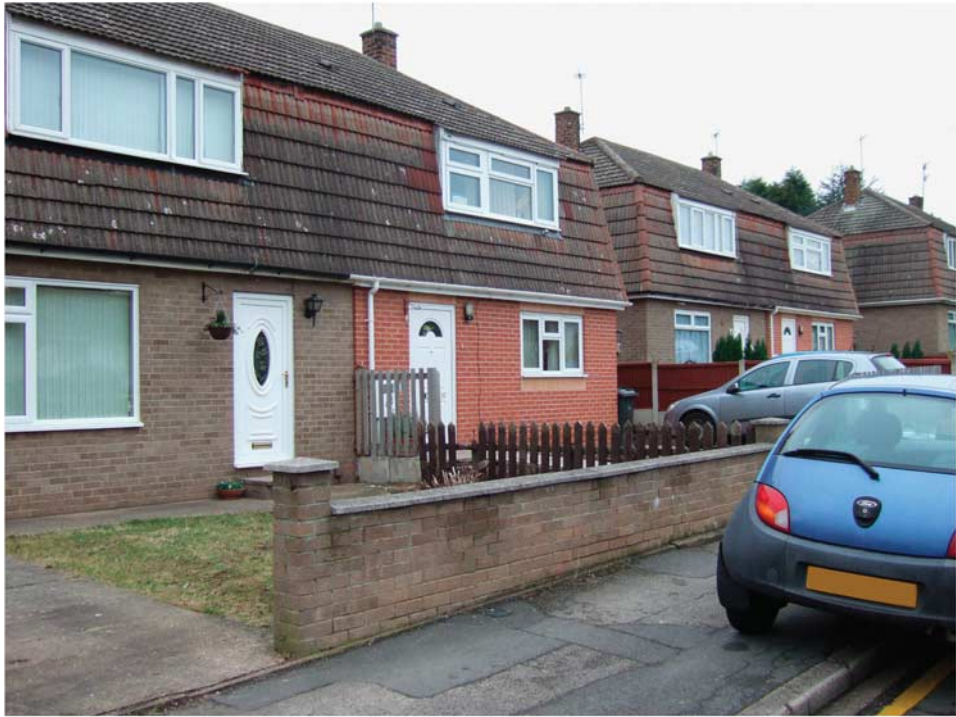
Figure 2: Once face-lifted with brick cladding and new UPVC fenestration, they can be made aesthetically attractive.
